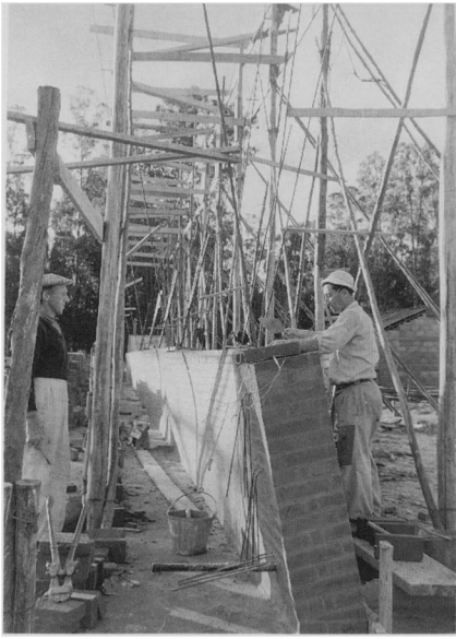
6 Church of Atlantida, wall under construction.
