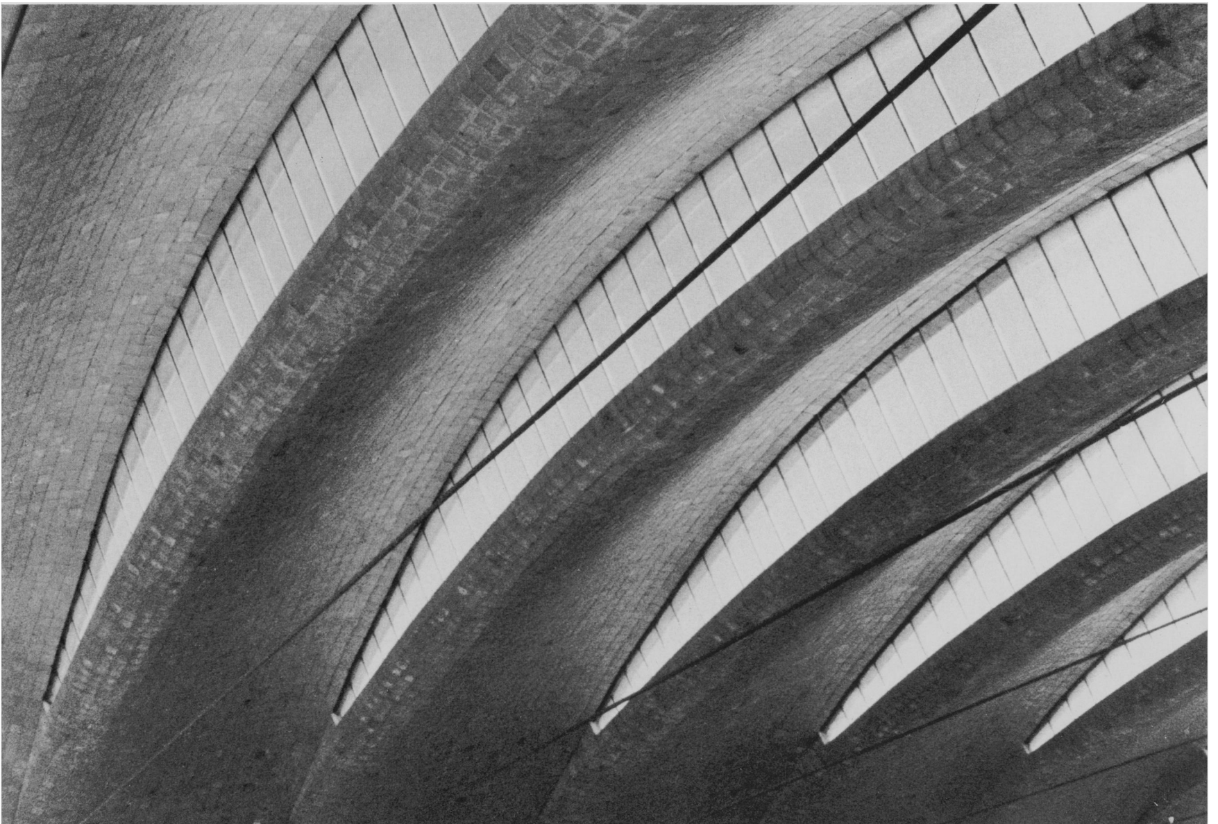
18 Warehouse, detail of clerestory lights.
